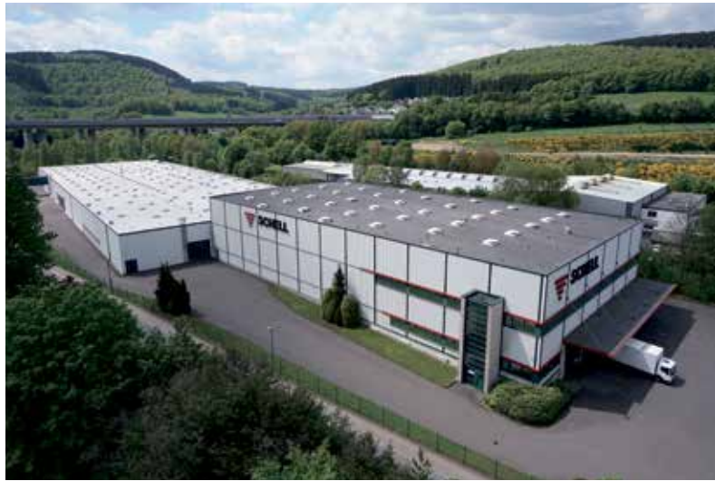
Plant 2 Production with logistics centre
